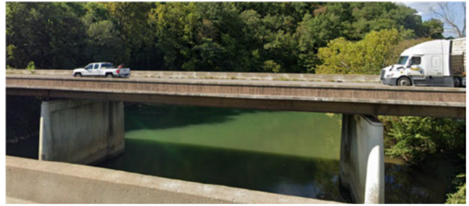
Figure 22 – Buffalo River Bridge on I-40 West in Humphreys County
